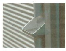
As water flows from the gutters it carries leaves and small pieces of debris. The Leaf Eater® incorporates a flow directional gutter outlet which directs the flow of water onto the face of the **primary screen**. The water washes over this screen which has a 6mm aperture and is set at an angle to the horizontal of around 45°. This angled screen is selfcleaning and forces the leaves and debris away allowing the water to continue through towards the **secondary screen**.
