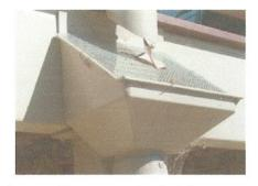
The Leaf Eater® can also be mid-mounted on a wall at a convenient height to make it easier to access for cleaning. When mid-mounting, the gutter outlet is discarded and the entry downpipe is cut at 45°, allowing 50mm clearance between the pipe and the primary screen.
