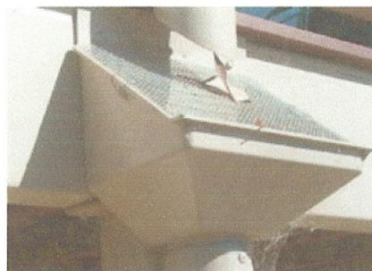
The Leaf Eater® can also be mid-mounted on a wall at a convenient height to make it easier to access for cleaning. When mid-mounting, the gutter outlet is discarded and the entry downpipe is cut at 45°, allowing 50mm clearance between the pipe and the primary screen.
